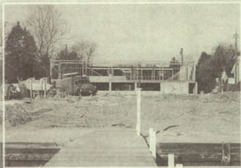
Rear view of new Clubhouse under construction.
