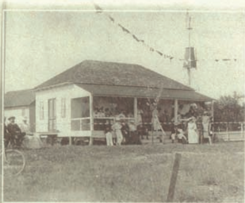
MRYC's first clubhouse, 1901 to 1904, was a former cyclists' rest stop/ice cream pavilion, located next to the old bridge, between Brielle and Point Pleasant, at Higgins Avenue.
