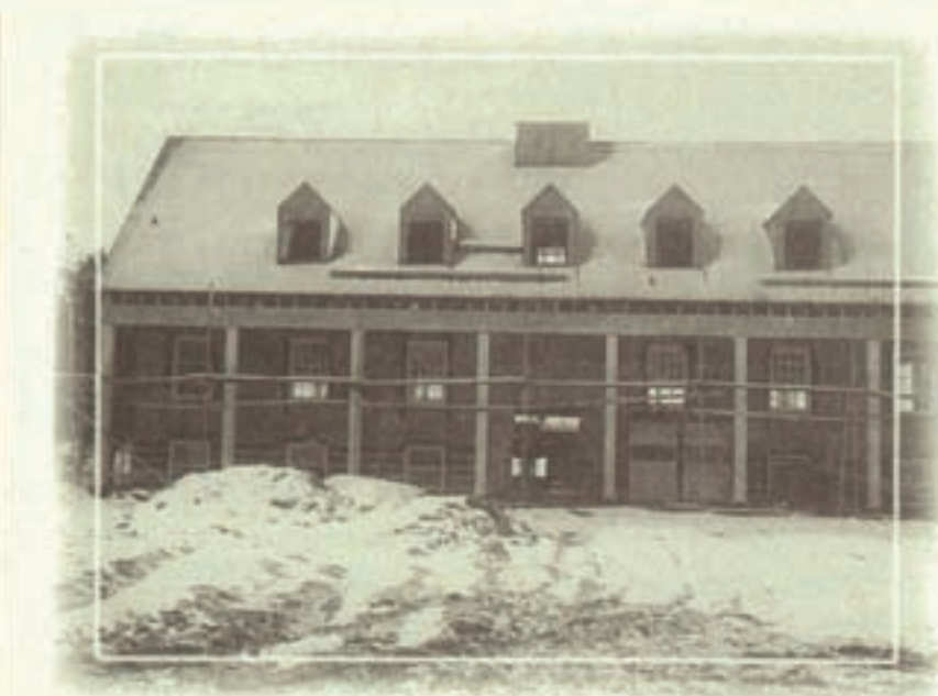
New Clubhouse under construction in the winter of 1962.
